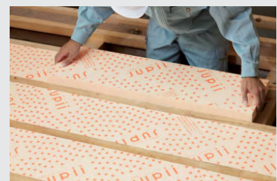
Jupii™ phenolic foam insulation panels for wood-frame houses
