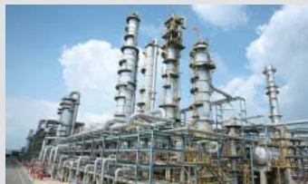
Propane-process acrylonitrile (AN) plant in Thailand
