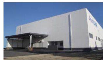
The second manufacturing facility at the Nagoya Pharmaceuticals Plant
