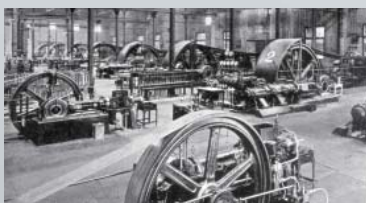
Part of the ammonia plant completed in 1923 (Nobeoka, Miyazaki, Japan)
