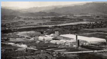
The Bemberg™ plant which started operation in 1931 (Nobeoka, Miyazaki, Japan)
