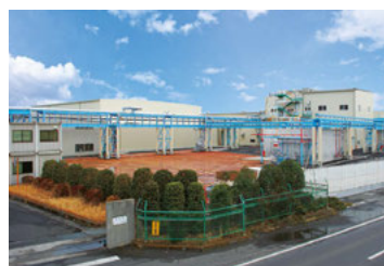
Plant for Neoma™ panels
