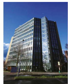
Asahi Kasei Europe's office building
