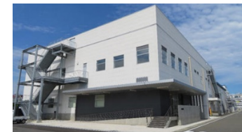
Planova hollow fiber spinning plant (completed Sept. 2019)
