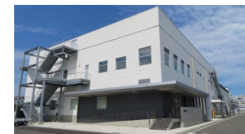
Planova hollow fiber spinning plant (completed Sept. 2019)
