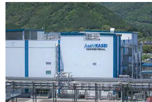
Assembly plant completed in May 2024
