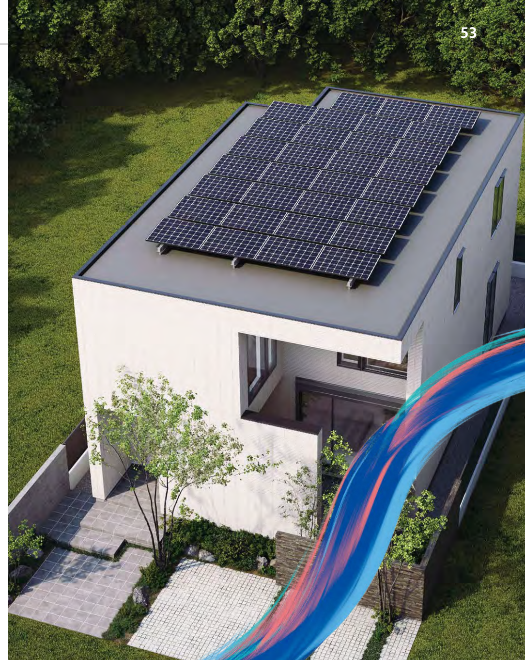
New "earth-tech" product to enable net zero CO 2 throughout the lifecycle of the home (Homes sector)
