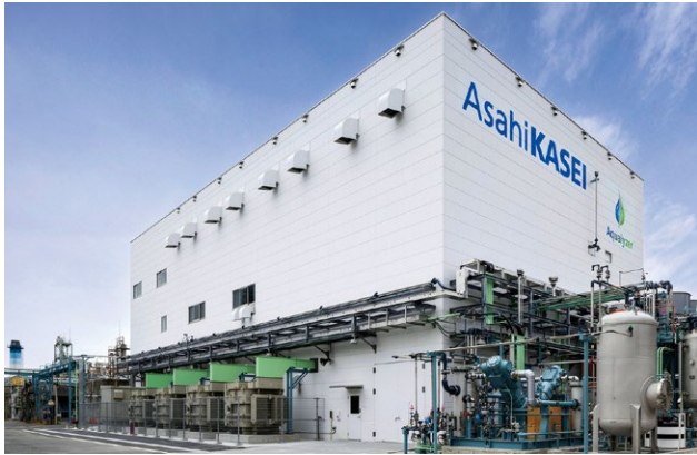
Alkaline water electrolysis pilot plant at the Kawasaki Works which began operation in fiscal 2024
