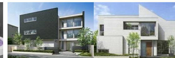
Hebel Haus unit homes Hebel Maison apartment buildings Providing long service life to reduce GHG emissions from component manufacture and construction
